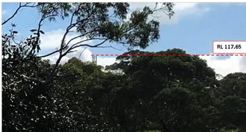
Optus Base Station at RL 117.65 visible above tree canopy. Photos taken from Seven Little Australians Park. The proposal seeks an increased height to RL 127.3 making it highly visible above the canopy.
