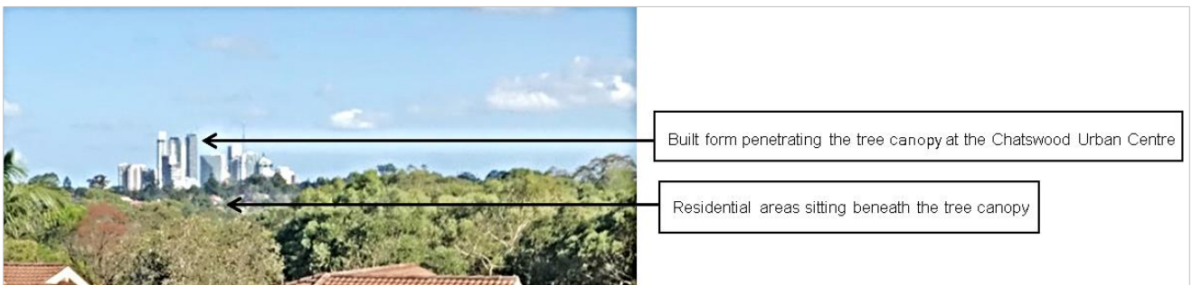
Ku-ring-gai's prevailing tree canopy character with dominant built form only to urban and local centres. (Photo taken from Lourdes site)
