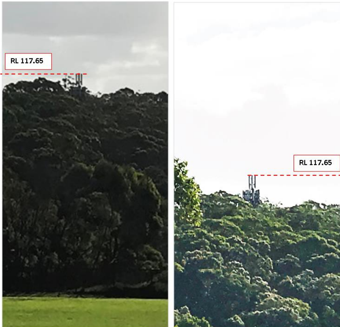
Optus Base Station at RL 117.65 visible above tree canopy. Photo taken from Lindfield Soldiers Memorial Park and oval. The proposal seeks an increased height to RL 127.3 making it highly visible above the canopy.
